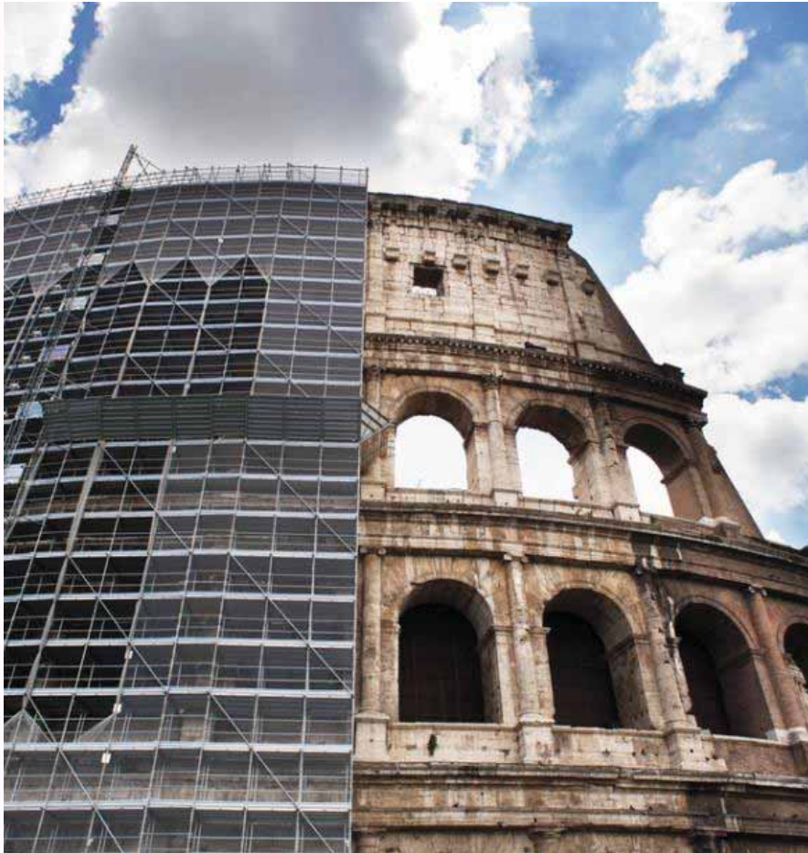
Recent restoration works on Colosseum (from Corriere della Sera, 14 July 2014)
