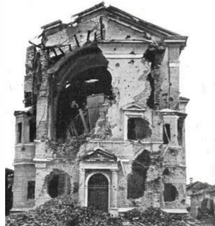
A church damaged during the I World War ; S. Andrea sull'Isonzo, Italy
