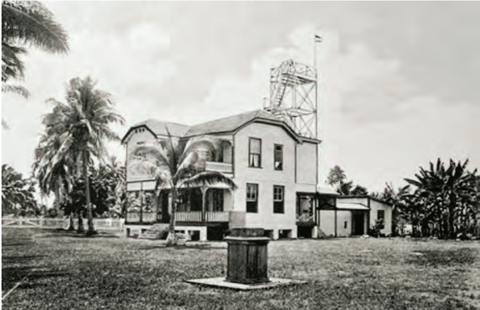
Observatory in Apia, Samoa. New service building, designed by Franz Linke and Fritz Stünzner, 1905. Photographer unnamed (Linke).
