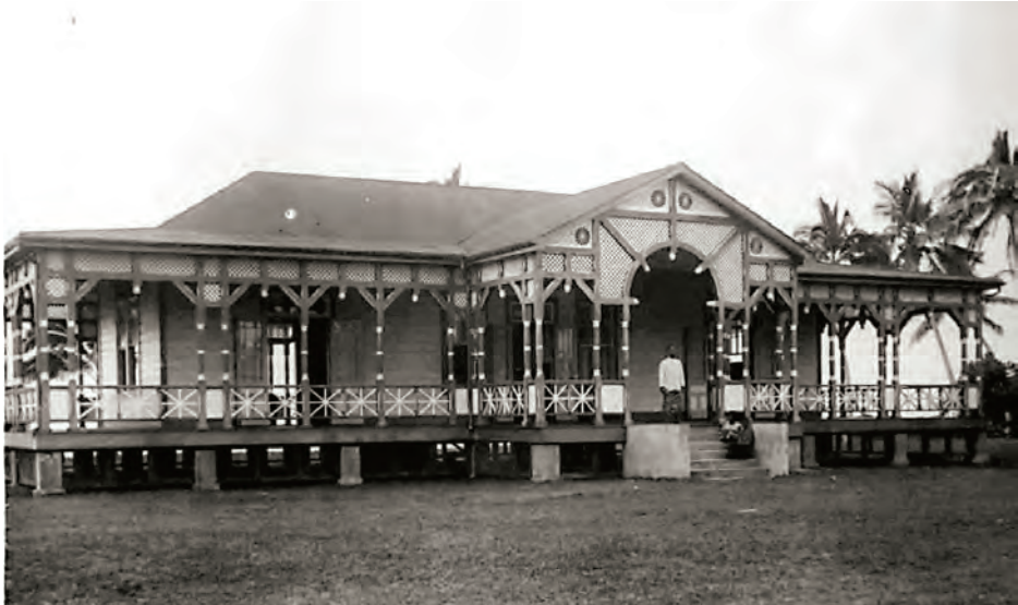
Albert Schaaffhausen: Building for the Samoan Self-Administration at Mulinu'u, Samoa, 1909 7101_3162_3412_0068 Koloniales Bildarchiv Frankfurt
