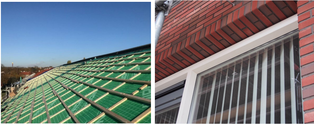
Figure 3: The installation of rood insulation and the renovated building envelope
