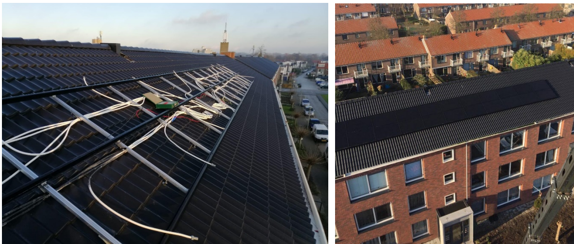
Figure 11: Installation of the PVT panels
