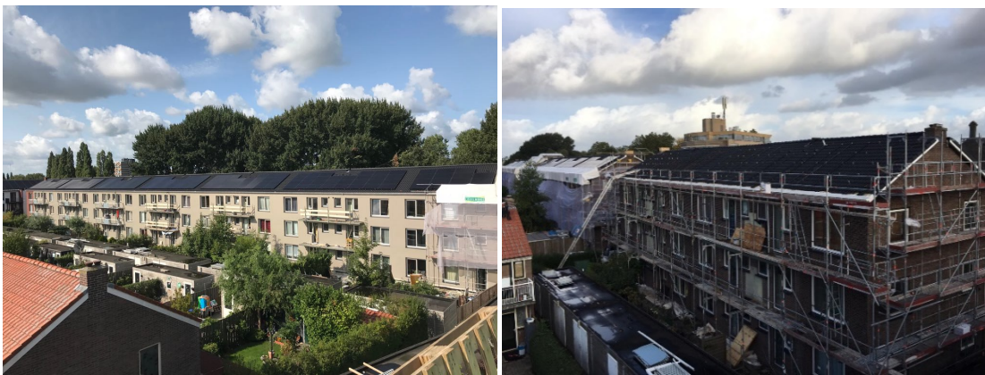
Figure 2: The buildings during renovation
